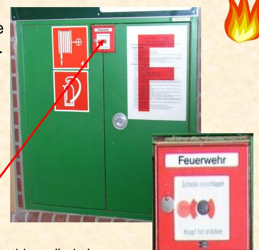
the buttons are protected by a thin walled glass
