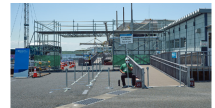
End of Line
