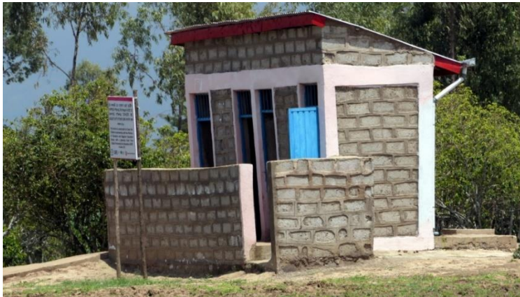
Fig. 11: Double VIP latrine blocks separated by gender were built in 17 of the 20 schools of the StC project in Sidama.
