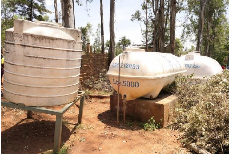
Fig. 10: Older 5,000 litre water storage tank from previous support and 10,000 litre tank connected to the local network (provided by the StC project in Sidama).
