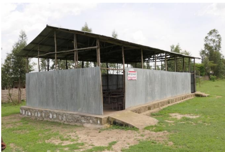
Fig. 9: Corrugated iron hangar built by the StC project in Boricha woreda for use as a canteen for school meals in Sidama.
