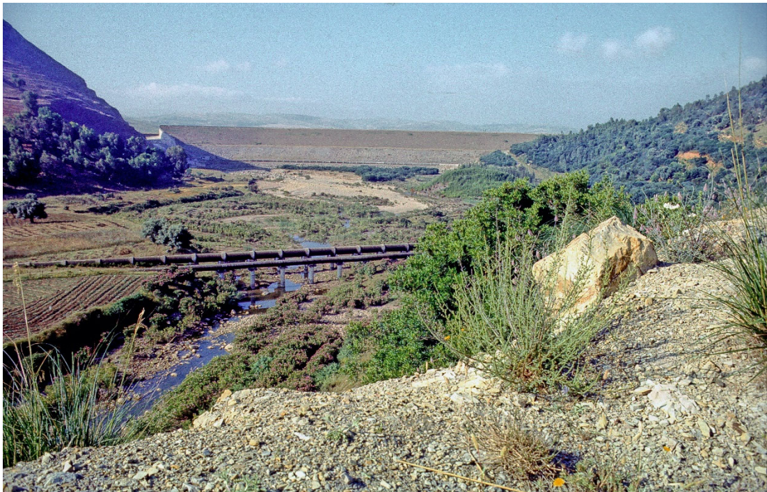
Fig. 10: The Bou Heurtma dam, feeding an irrigation perimeter of almost 20,000 hectares (the picture shows the main water pipeline).
