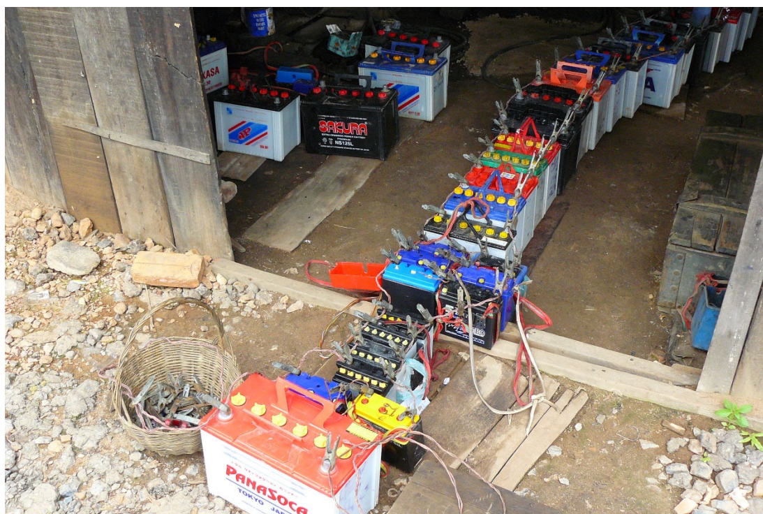
Fig. 18: Where villages in Cambodia are not connected to the central power grid, poor households in particular have to spend a lot of money for the "luxury" of a minimal power supply (here: private charging station for car batteries)
