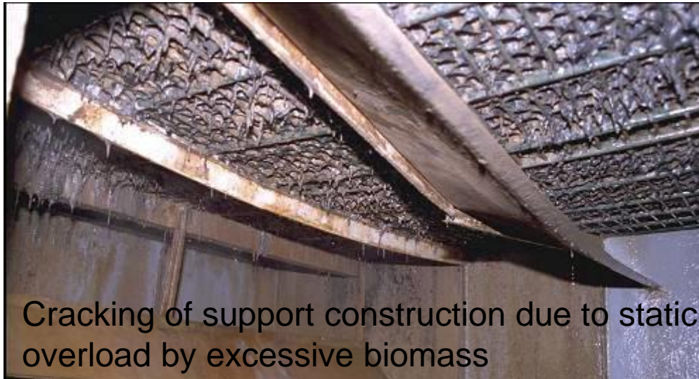
Heat exchangers with massive biofouling
