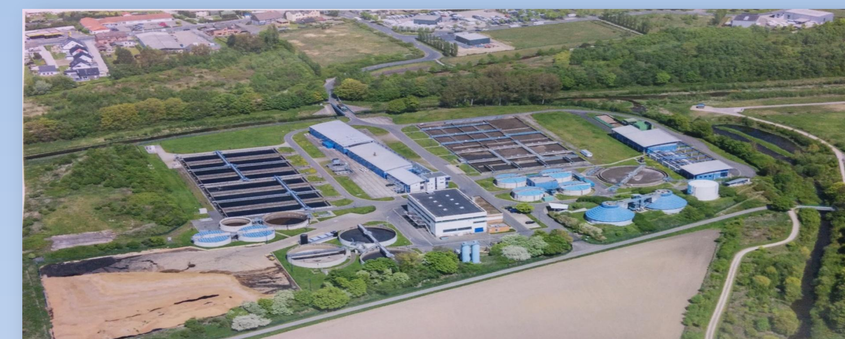
Figure (3): Wastewater treatment plant in Kamen
