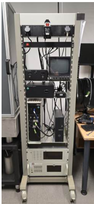
Figure 3.2: SPM controller, HEB (electronics head box), control computer (old and new), as well as the SPM components for AFM measurements in a 19-inch laboratory rack.
