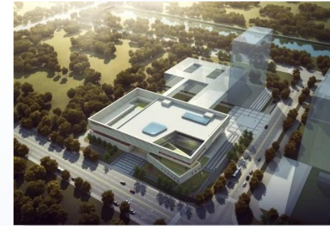
Proton Center (under construction)
