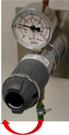
1. At first turn the wheel for the nitrogen which is located on the wall behind the SEM in clockwise direction until you see the green marking. The nitrogen is required for gas flooding of the air-lock.
